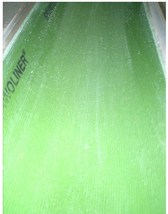
Figure 16: Sample item B1003-1.2 after the abrasion test with 200,000 load alternations
